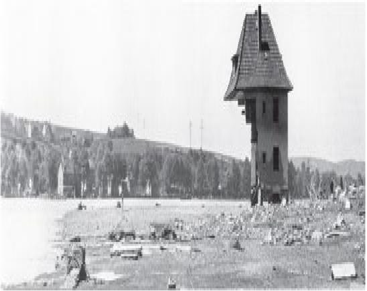
Destruction at Neheim, six miles downstream from the Möhne.
