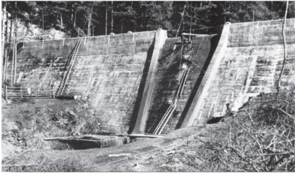
Nant y Gro dam in Wales. Tests here in July 1942 proved that the German dams could be destroyed with far less explosive than had originally been thought.
